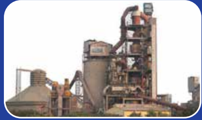
CEMENT PLANT MACHERLA
