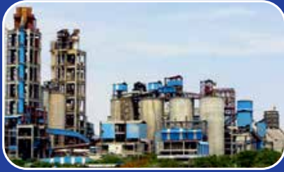
CEMENT PLANT MUKTYALA
